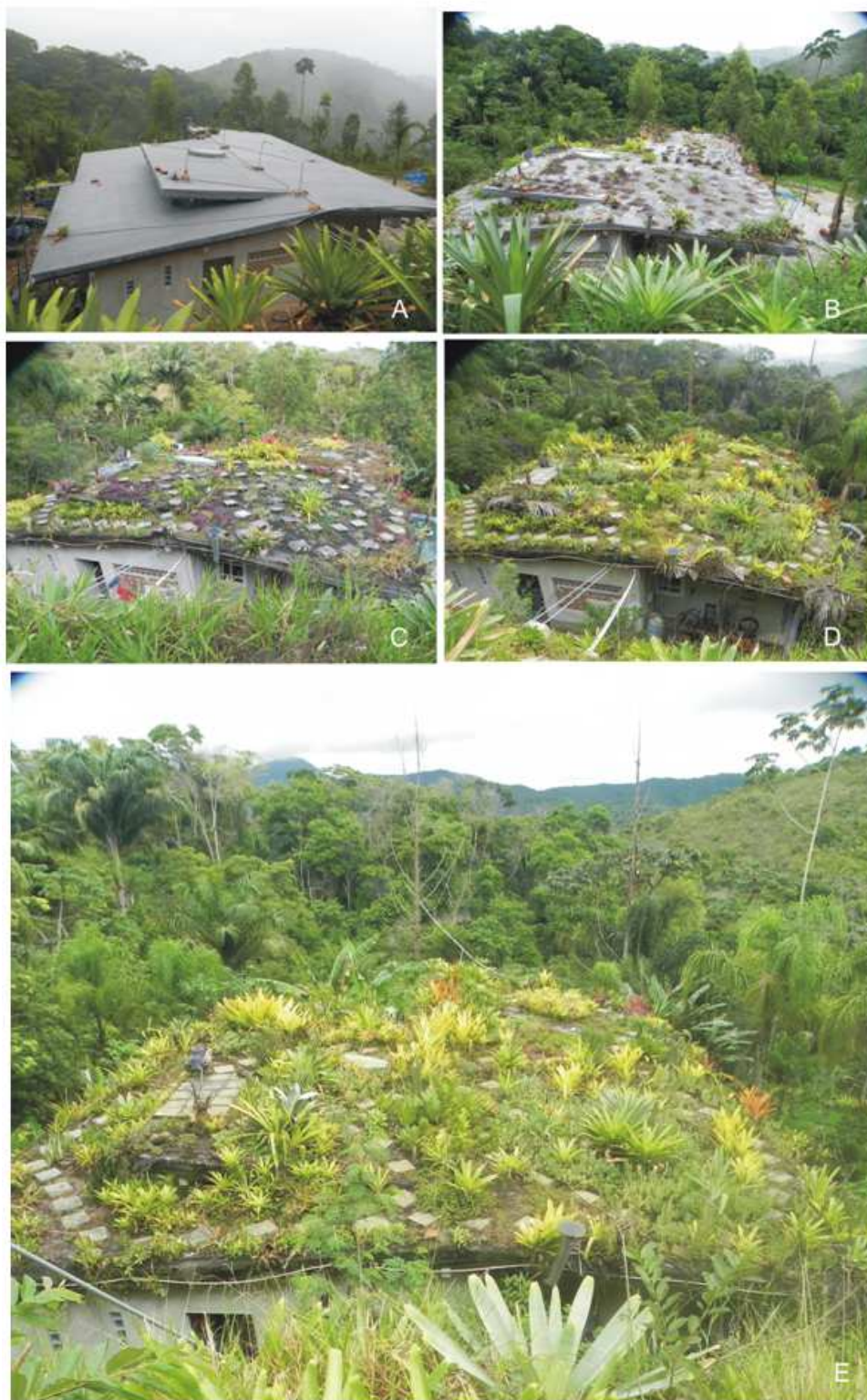
Fig. 7: Cronosequence of a tropical greenroof installation in Southeastern Brazil. A. Greenroof with three layers (thin geotextile, waterproofing membrane and thick geotextile) recently installed without vegetation-December 2012. B. Early planting of tropical species-March 2013. C. Steady clonal growth-October 2013. D. Established artificial community fully covering the roof area-May 2015. E. Artificial tropical greenroof community that has become stable on the long term-March 2016
