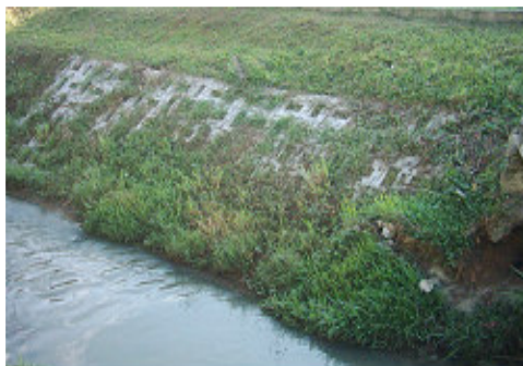
b. Right bank with side slope of 1 (V) : 1.5 (H)
