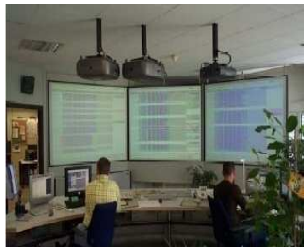
Fig. 2. Central Control Room (IKCO's CCR)
