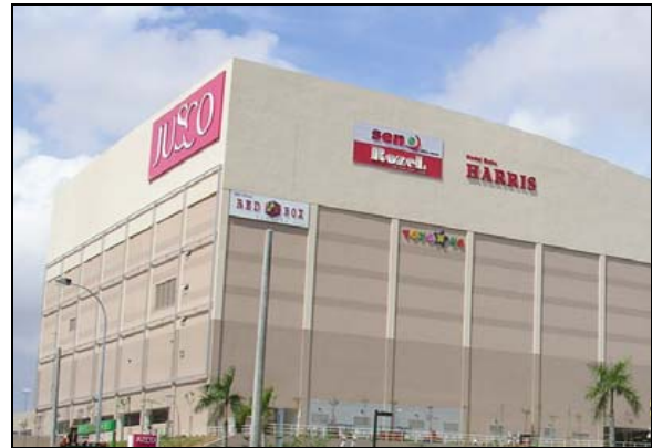
Fig. 1: Precast concrete structure-AEON Jusco Tebrau City, Tebrau, Johor Bahru
