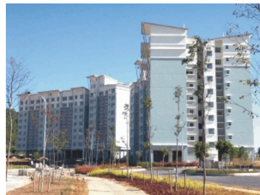
Fig. 3: Precast concrete structure-AIMST, Kedah
